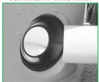
STEP 1: Bevel pipe. Clean connector. Clean pipe of dirt & debris.
