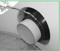
Attach proper size clamp beside o-ring then center pipe in connector and VERY **IMPORTANT** tighten clamp with torque wrench to 60 inch pounds.
