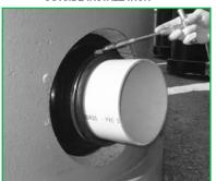
When installing a Z-LOK connector in the outside the manhole position pull pipe back out after inserting so the connector flips outward, then VERY IMPORTANT center pipe in connector and tighten the take down clamp to 60 inch pounds with a torque wrench.
